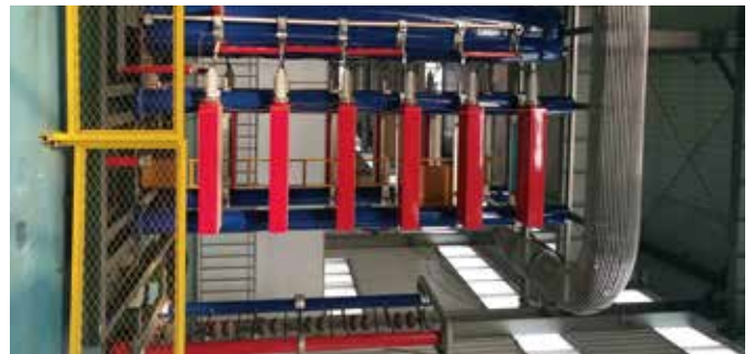
Lightning impulse voltage generator
