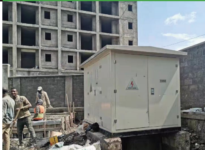
▲ Ethiopian box transformer installation site
